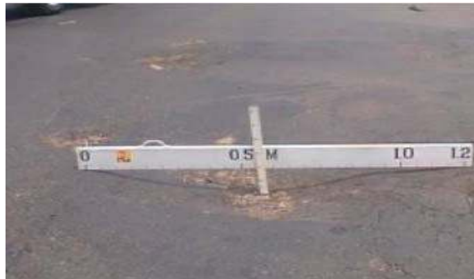
Gambar 2.5 Amblas ( Depression ) (Sumber: Bina Marga, 1983)
