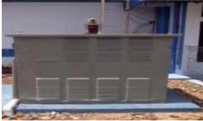
Gambar 2.14 Neutral Grounding Resistance (NGR)
