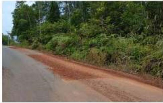
Gambar 2. 5 Tambalan (*Patching and Utility Cut Patching*)
