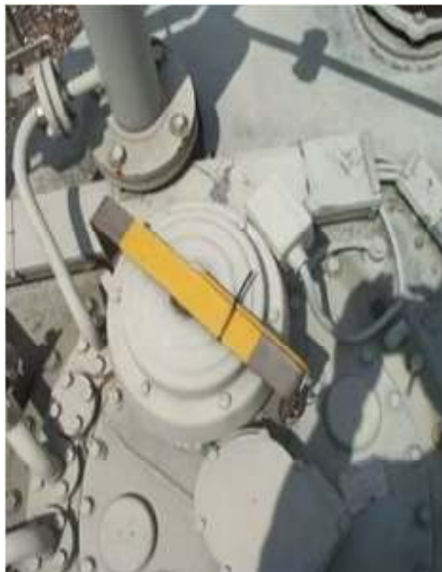
Gambar 2.17 Rele Sudden Pressure
