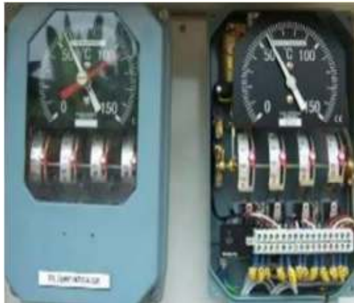
Gambar 2.18 Rele Thermal
