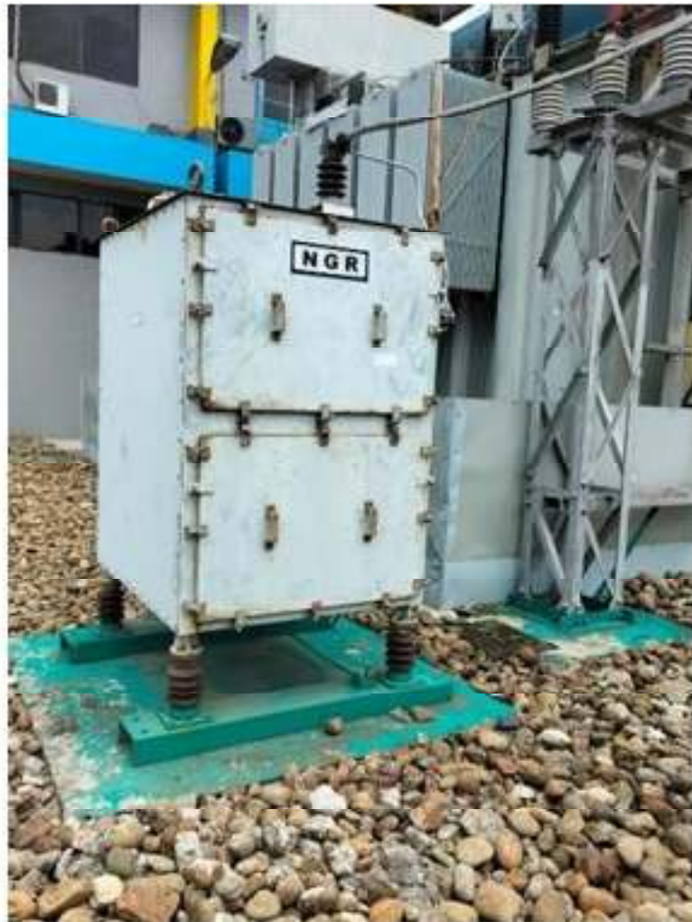
Gambar 2.19 Neutral Grounding Resistant (NGR)
