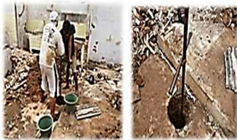
Gambar 2. 6 Bore Pile Manual
