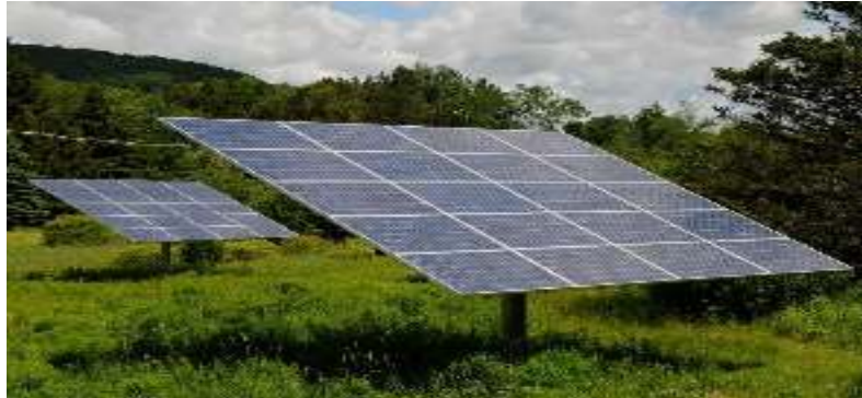
Gambar 2.6 Solar Tracker Dual-axis
