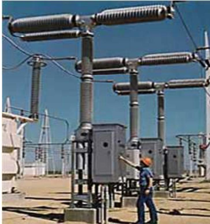
Gambar-2.9. SF6 Gas Circuit Breaker
