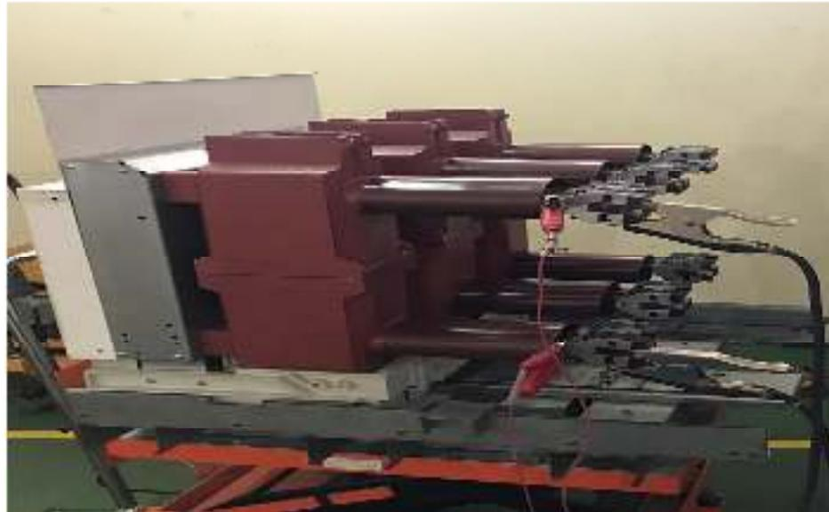
Gambar 3.9 Vacuum circuit breaker gardu induk Binjai
