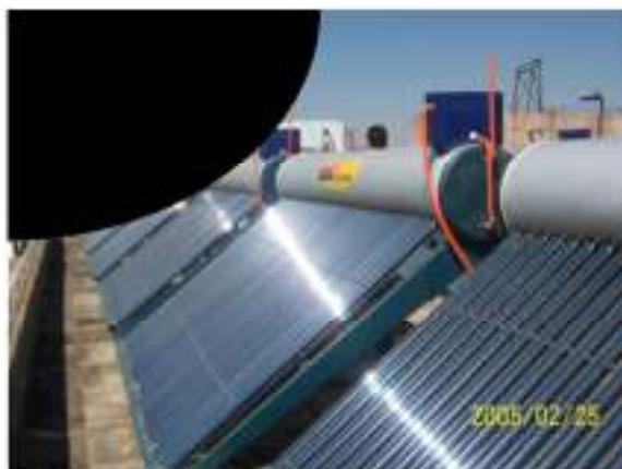
Gambar 2.4 *Solar Water Heater*
