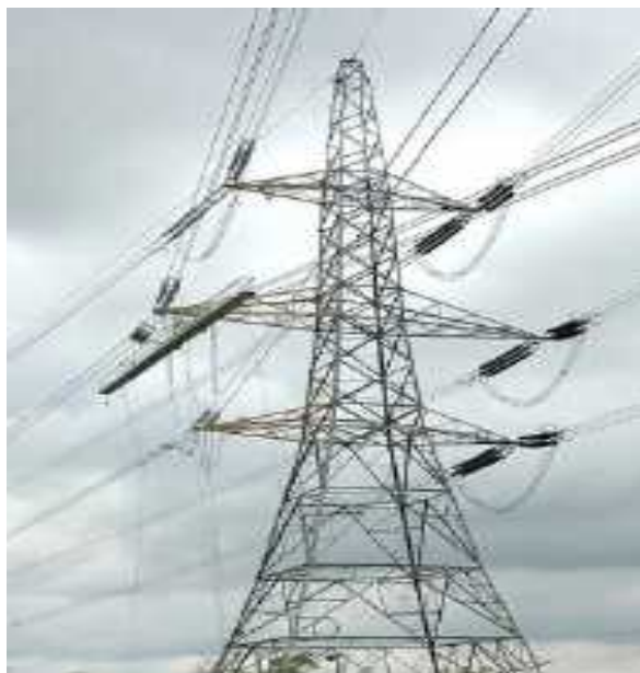
Gambar 2-8. Tension Tower.
