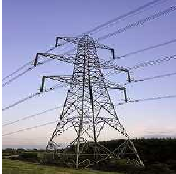
Gambar 2-7. Suspension Tower.
