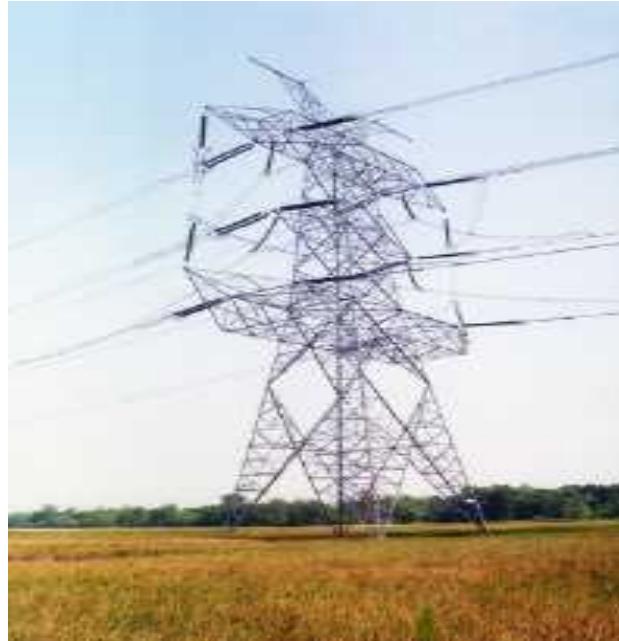
Gambar 2-9. Transposition Tower.
